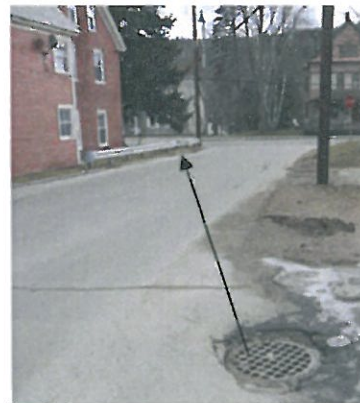
E Drop Inlet & Culvert Path (Facing South)
