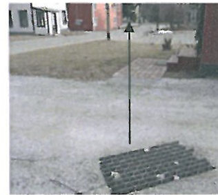
D Catch Basin Structure & Culvert Path (Facing South)
