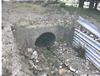
B Culvert Inlet w/ Headwall (Facing South)
