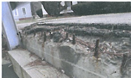
O Exposed Steel in Bridge Deck (Facing South)
